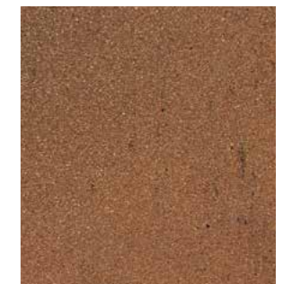
LIGHT RUST (TMD 52)
